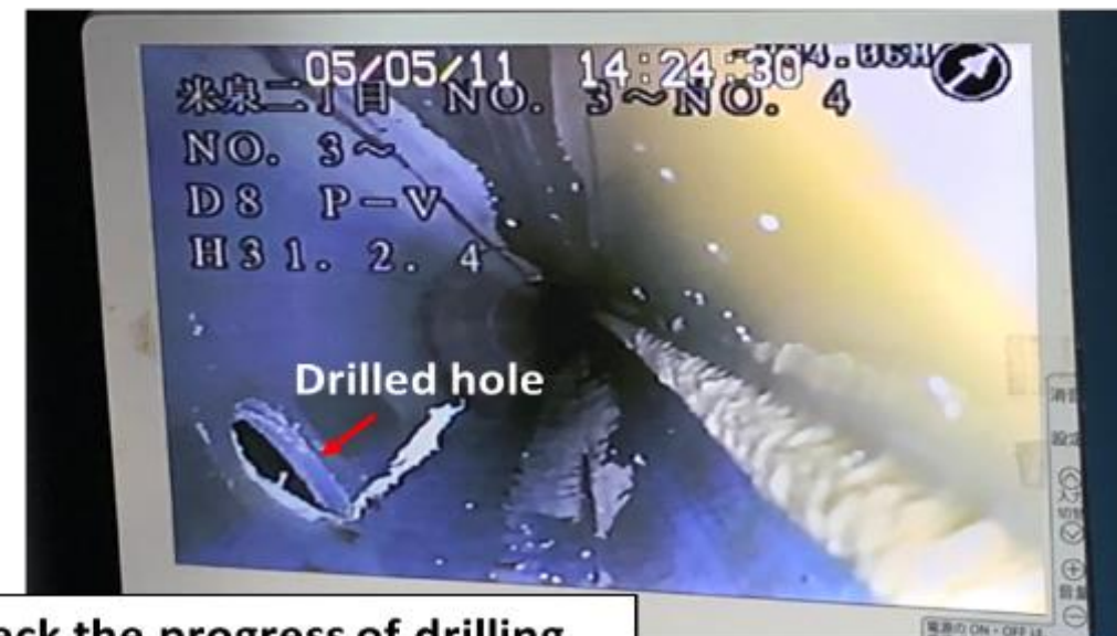
Using a pipe camera to check the progress of drilling
