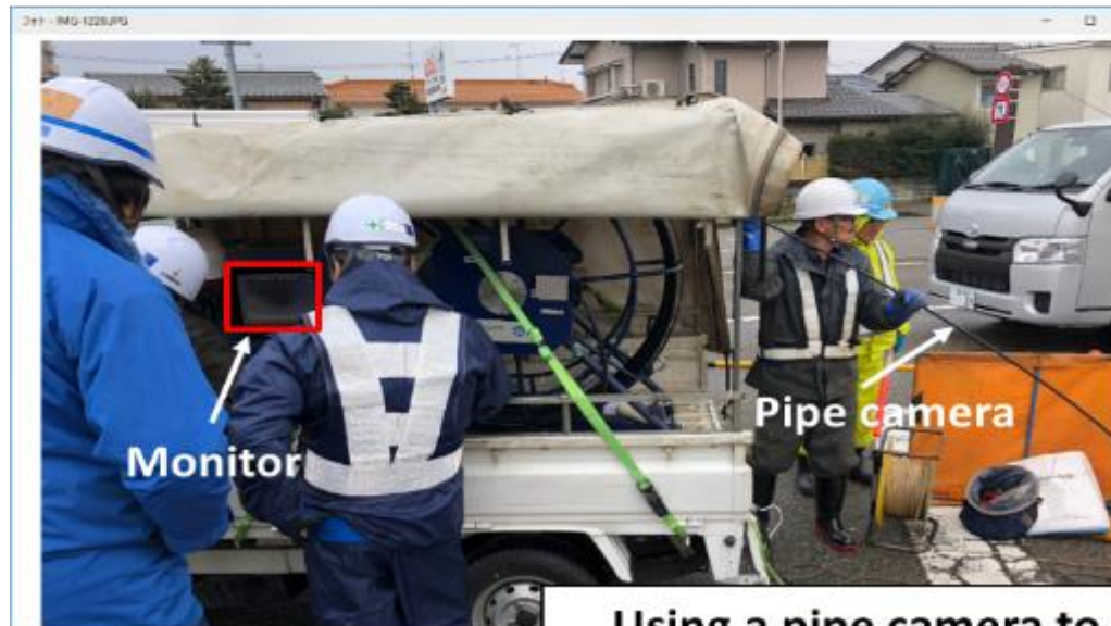
Using a pipe camera to check the progress of drilling
